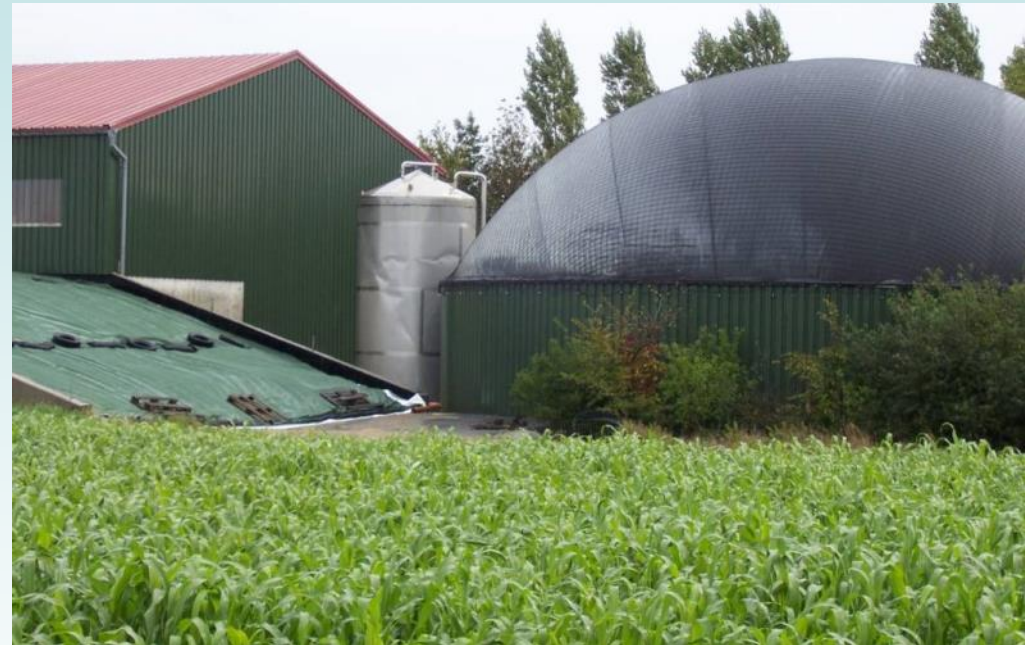
Biogas plant (Bavaria)
