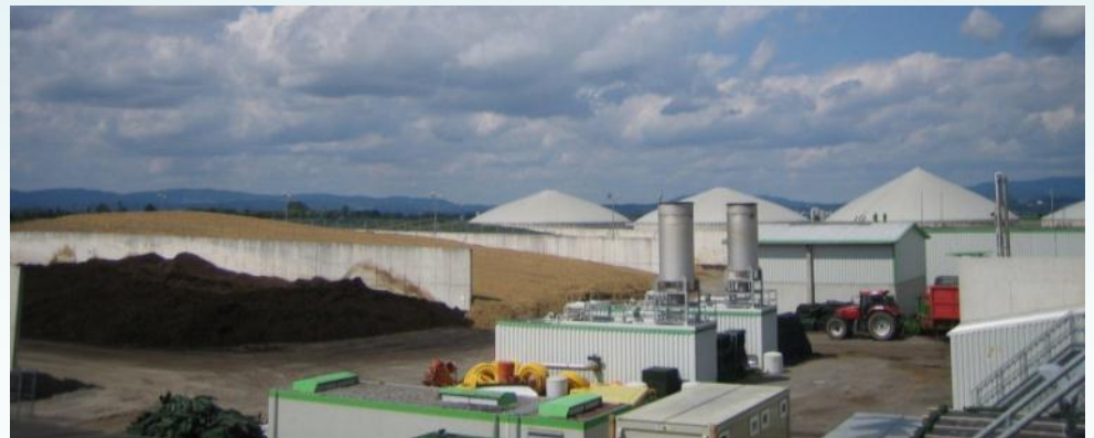
Biogas plant (Bavaria)
