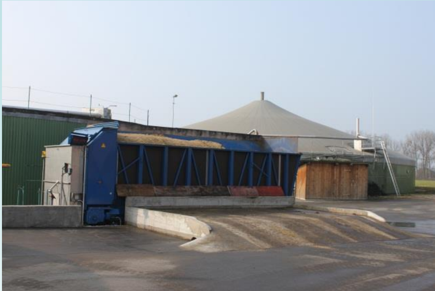
Biogas plant (Bavaria)
