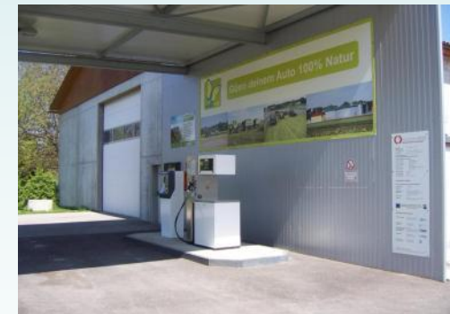
Biomethane filling station (Bavaria)
