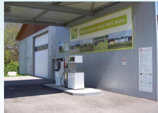
Biomethane filling station (Austria)
