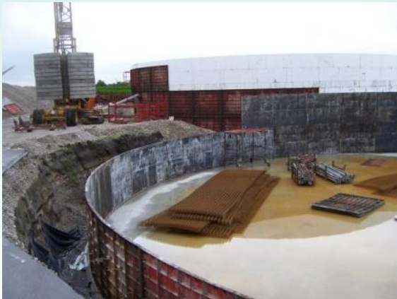
Concrete fermenter construction (Bavaria)
